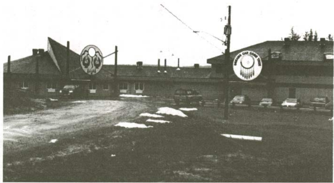
IMPRESSIVE AND PRACTICAL, the Mattagami FN community complex stands out as an achievement that you can't miss. The Complex houses administration and all community services and features a 10,000 square foot hall/gymnasium.
