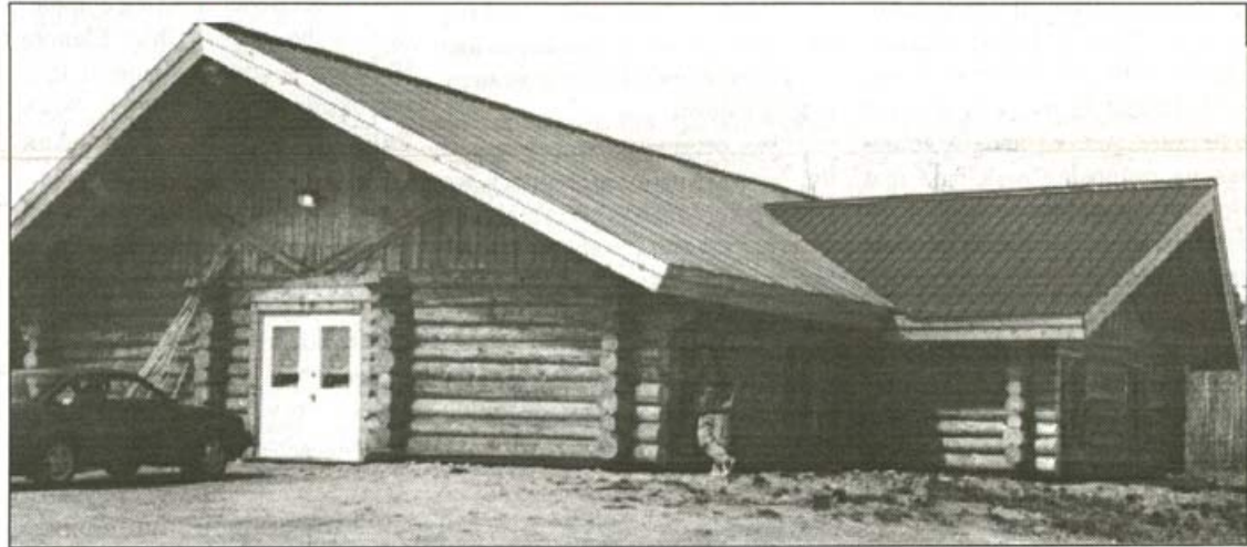
COMMUNITY PRIDE was given a big boost in Matachewan First Nation with the completion of the Matachewan First Nation Community Complex. Here we see Fabian Batise, Matachewan FN Band Administrator and Councillor at the 3,600 square foot, log complex.
